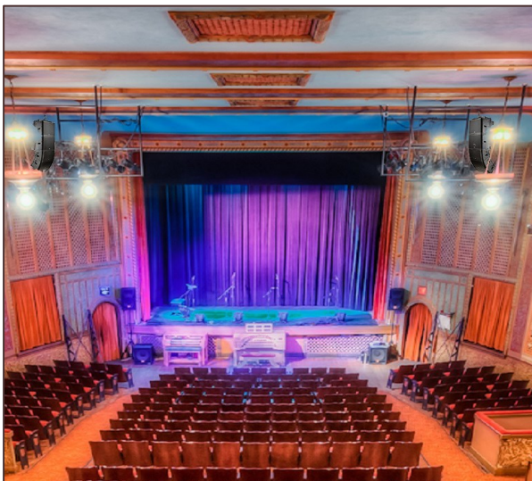
Line Array Speakers flown from the ceiling instead of floor speakers
